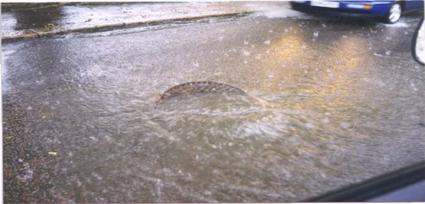
Figure 8 Flooding and floating manhole covers
